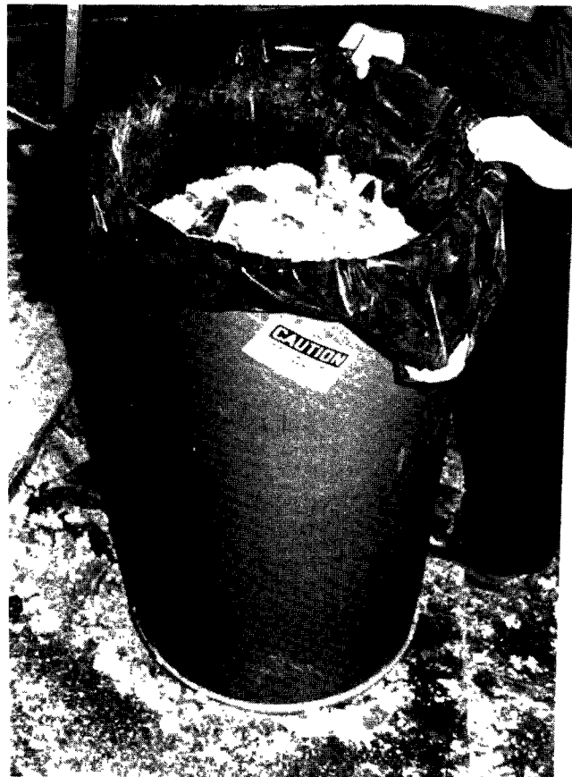
Figure 10. Plastic-lined cardboard container with asbestos waste.
